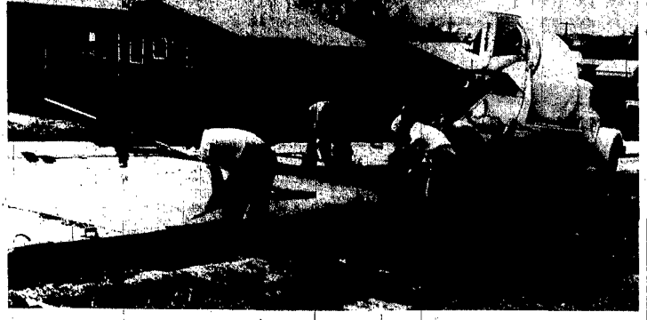
FIRST MAJOR PAVING work for this summer was completed this week with the finishing of Walnut street from Ninth to Tenth. The second phase is now underway with the paving of Ninth
